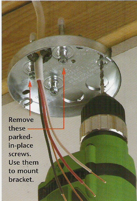
FBS405 Steel Fan/Fixture Box with Bright, Clean Finish
