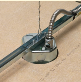
4 Cable pulled through cable connector (not supplied).
