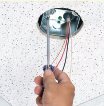
4 Remove captive screws (shown above). Use them to install the fan or fixture per manufacturer's specifications, NEC and all local electrical codes.
