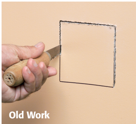
1 Position ONE-BOX adjacent to stud. Use box as template to cut hole.
