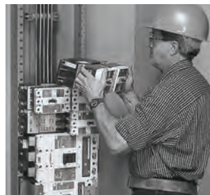
Panelboard Installation
