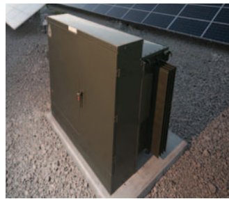
Medium voltage step-up transformer
