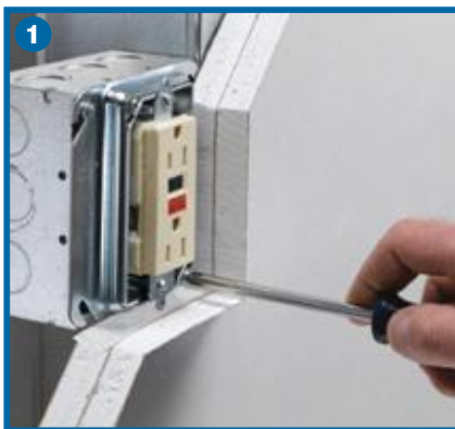
Loosen... The two adjustment screws located on opposing corners of the mud ring.
