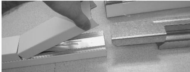
4. Slide TPP Extender into 25DTP-4 Tele-Power Pole.
