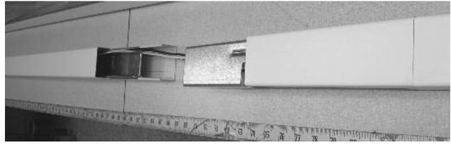
2. Remove the 8" [203mm] cover from the top section of the Tele-Power Pole.
