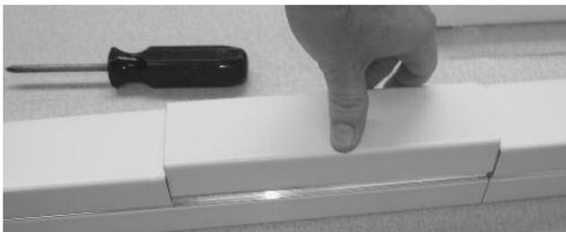
1. Line up Tele-Power Pole Extender with top of 25DTP-4 Tele-Power Pole with the longer sleeve on the same side as the 8" [203mm] top cover of the existing pole.
